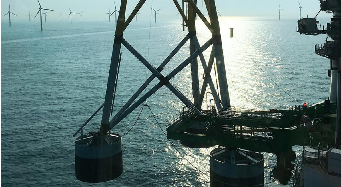
*The first of 20 offshore wind turbine foundations using suction bucket technology is lifted off the barge and ready to be lowered to the seafloor and penetrated by suction into the seabed.*
