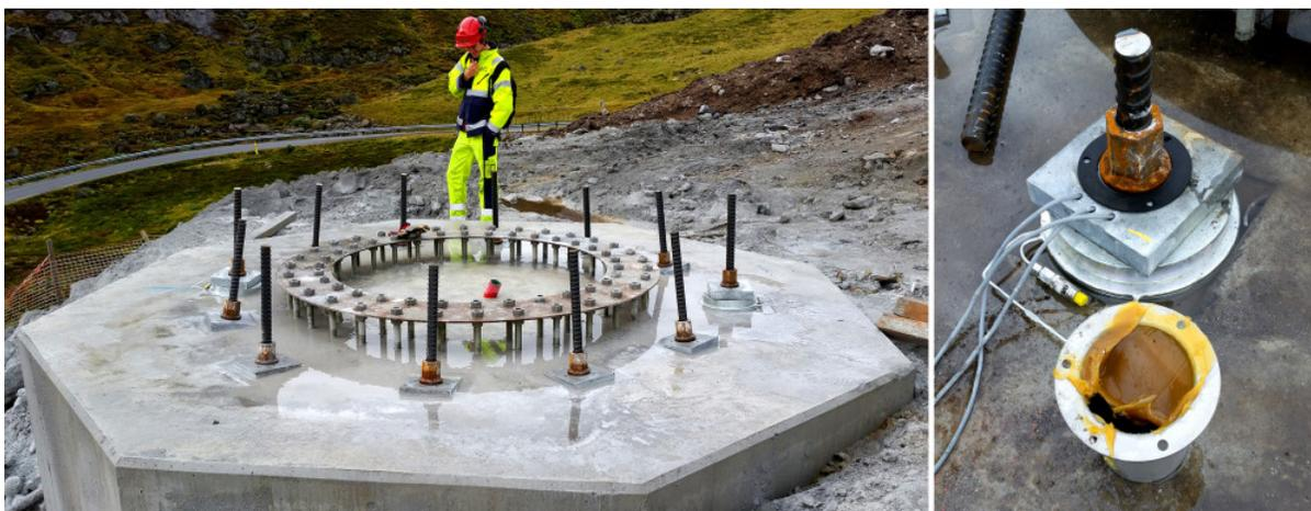
*Left: The pylon foundation with 12 rock anchors, and cast foot bolts for connection to the tubular towers. Right: Anchor head with load cell, load distribution plate, locking nut and protection lid filled with grease. (Photo: NGI).*
